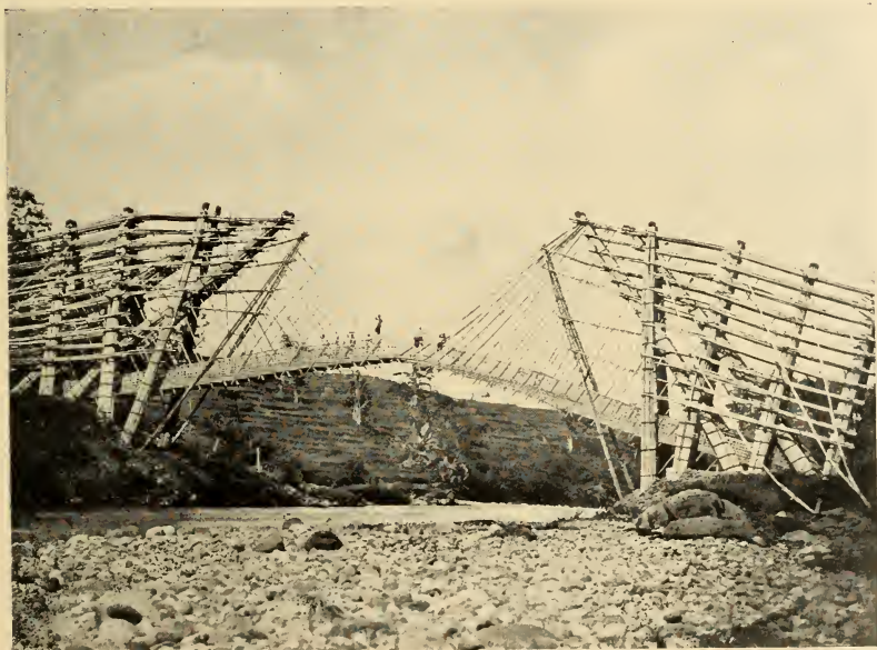
NATIVE ENGINEERING : A BAMBOO CANTILEVER BRIDGE.
